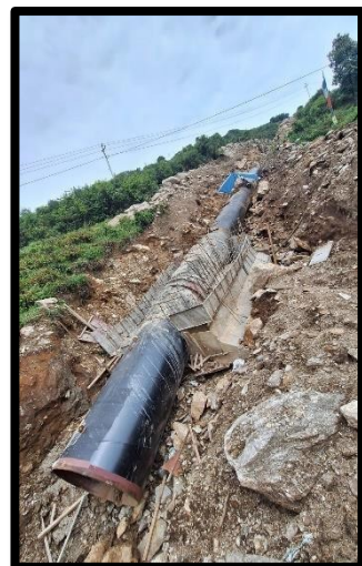
Penstock Pipe Erection
