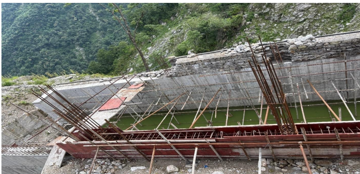
Figure 27: Construction of cooling pond along tailrace
