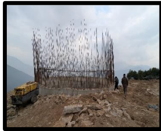
Surge Tank Backfilling
