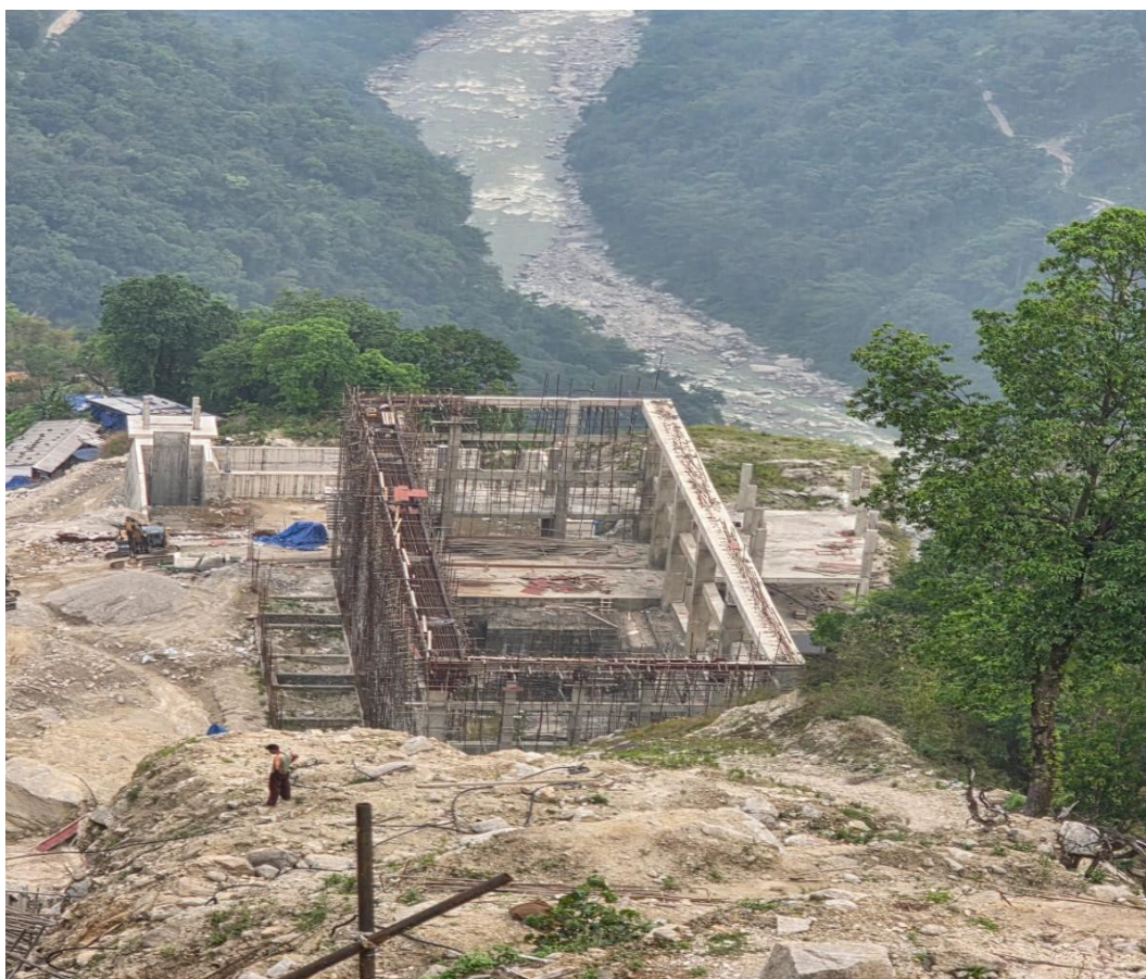
Figure 23: Bird's eye view of the powerhouse
