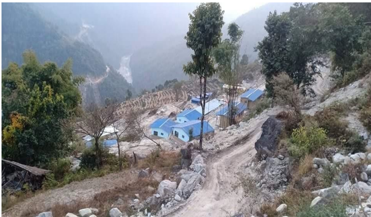
Figure 6: Employer's residential camp at Powerhouse
