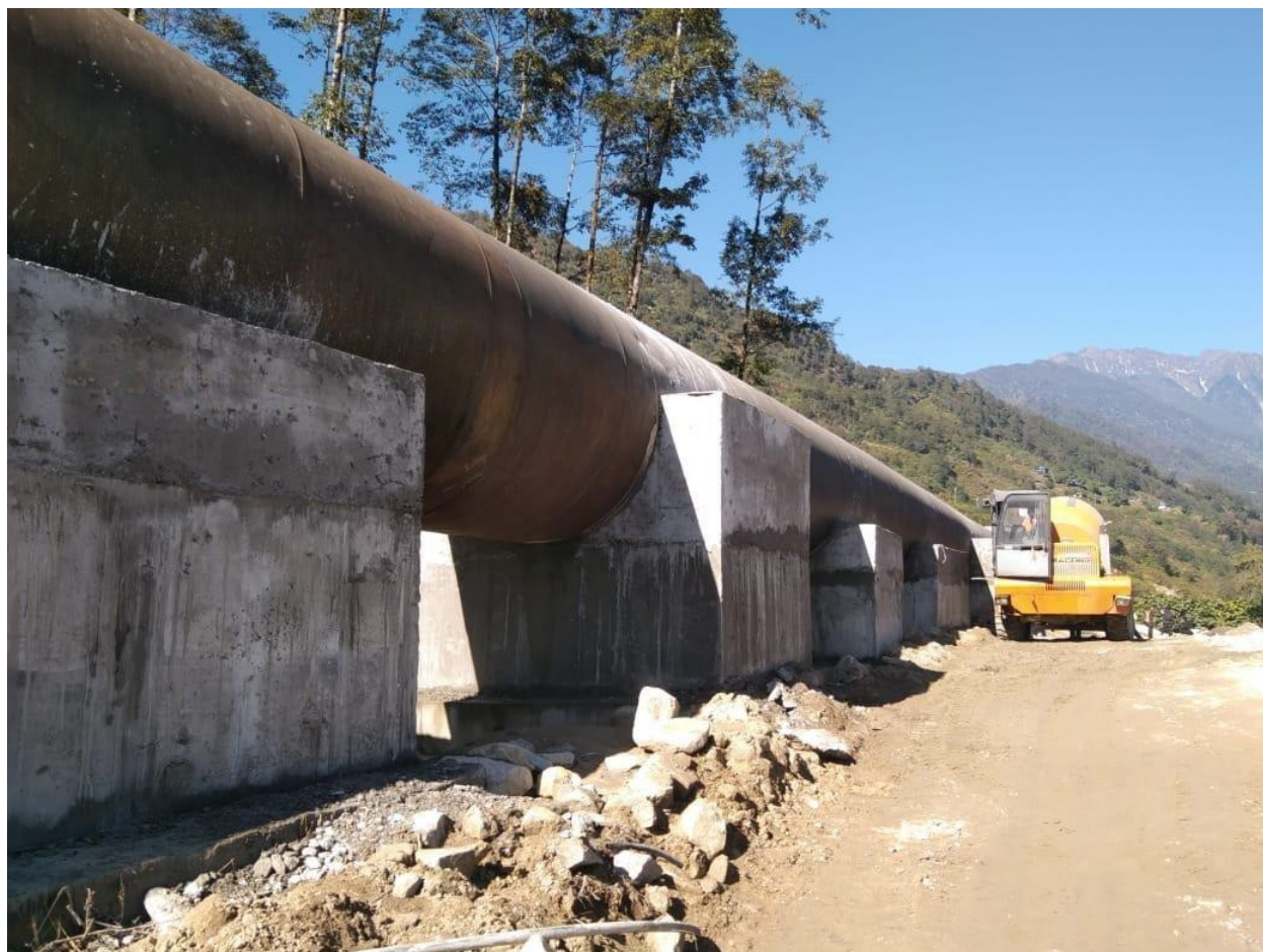
Figure 16: Jacketing works in support pier at headrace pipe alignment
