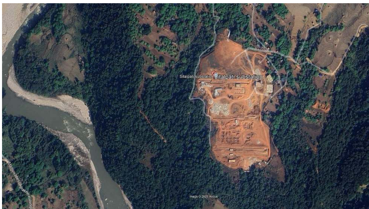
Figure 32: Sitalpati substation (NEA Project)
