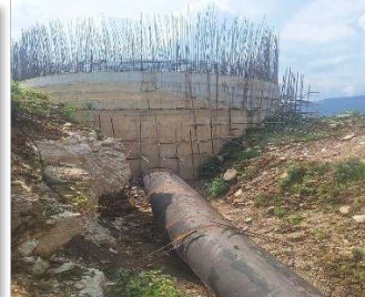
Penstock side view of surge tank
