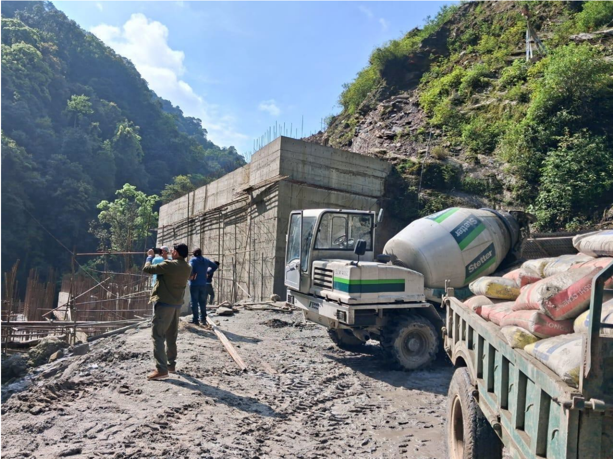
Figure 9: Undersluice, intake view
