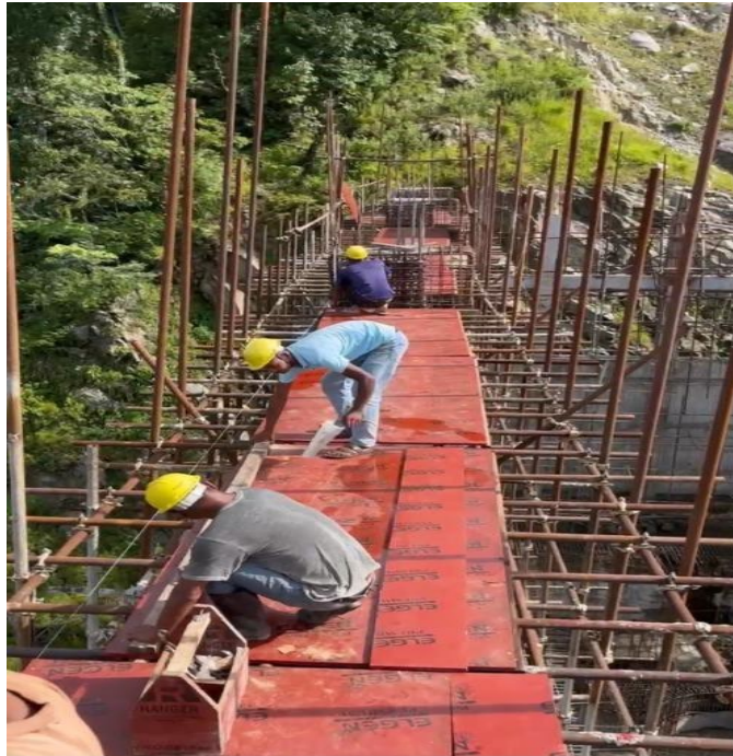
Figure 24: Preparation of Concreting at corbel beam level
