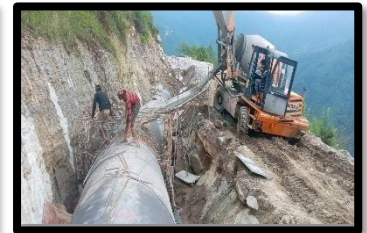
Anchor Block construction
