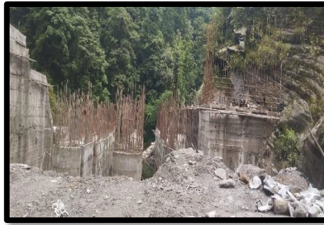
Under-sluice Concreting
