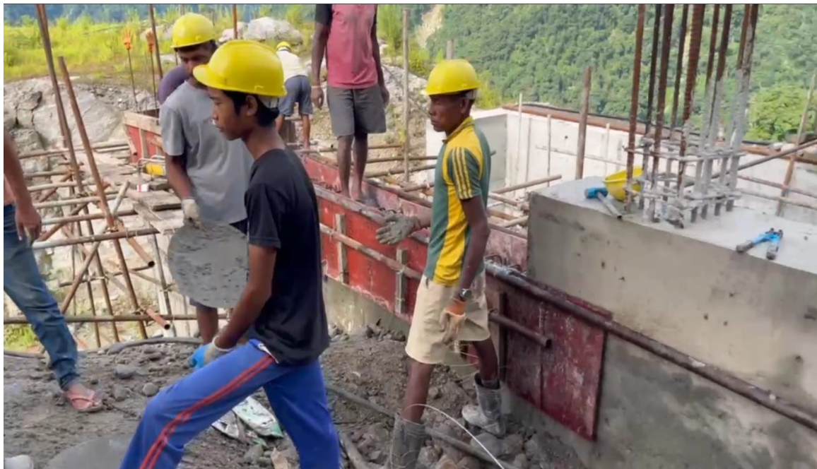
Figure 25: Ongoing construction of top slab for the cooling chamber
