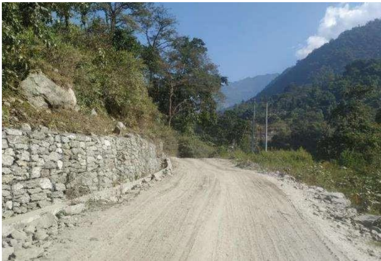
Figure 3: Gabion wall construction at access road from Arun River to Powerhouse Area
