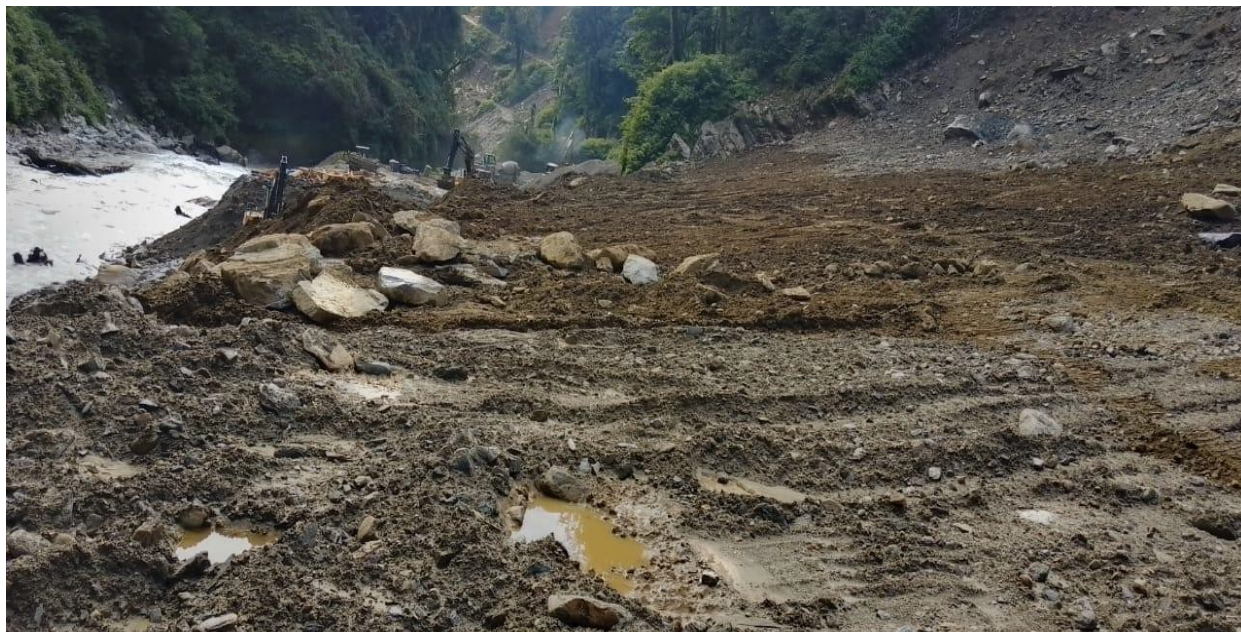
Figure 10: Excavation on pondage area
