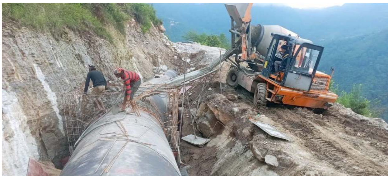
Figure 15: Construction of anchor block at headrace pipe alignment
