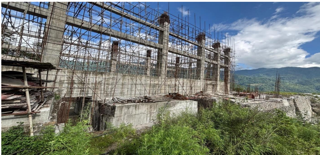
Figure 26: Construction of tailrace
