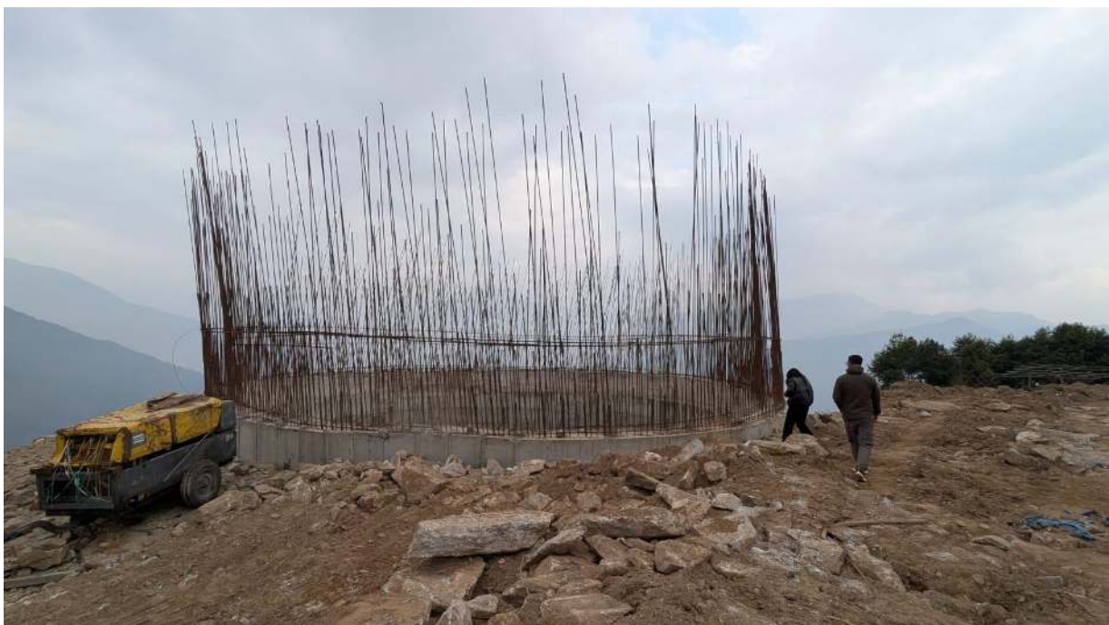
Figure 17: Backfilling of surge tank
