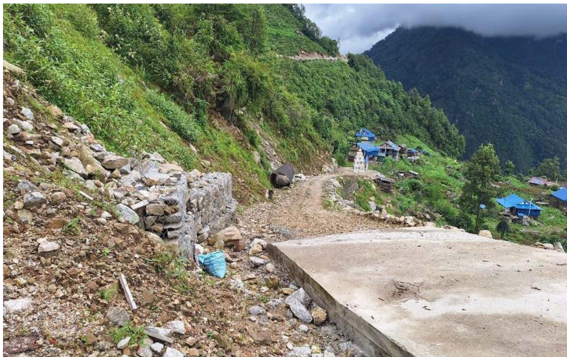
Figure 33: Excavation of road at Yangluwa
