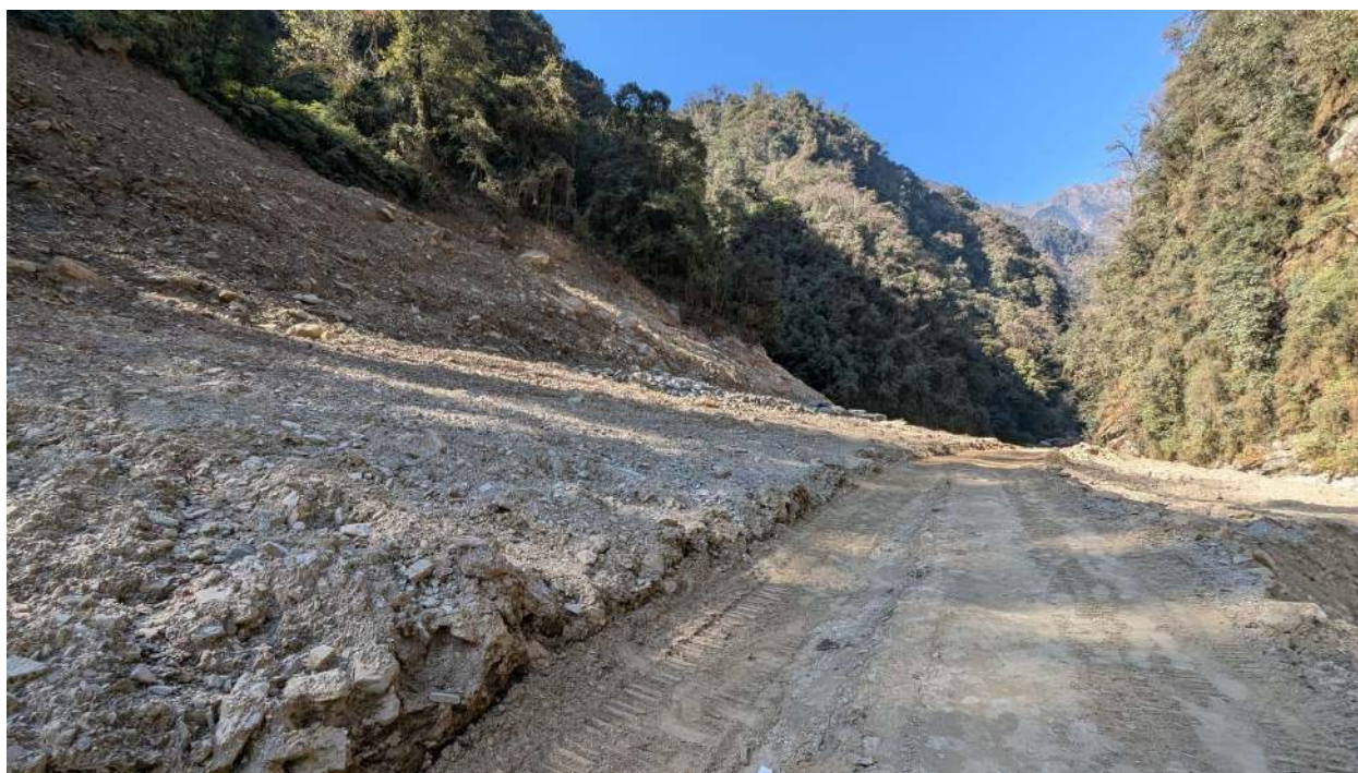
Figure 11: Slope cutting on pondage area
