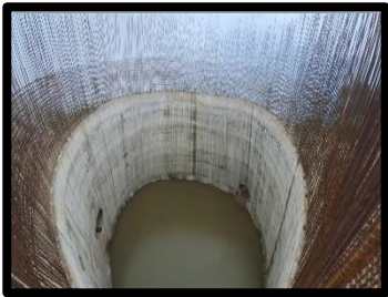
Surge Tank Inner View
