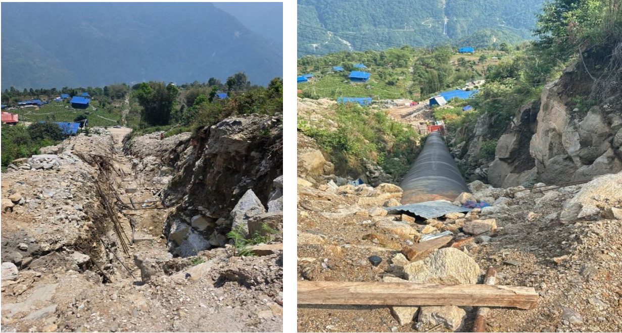
Figure 22: Construction of penstock pipe and site preparation
