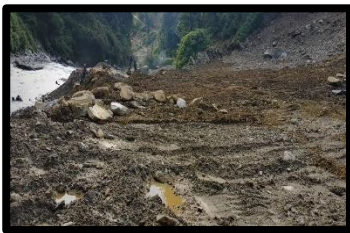
Pondage area excavation
