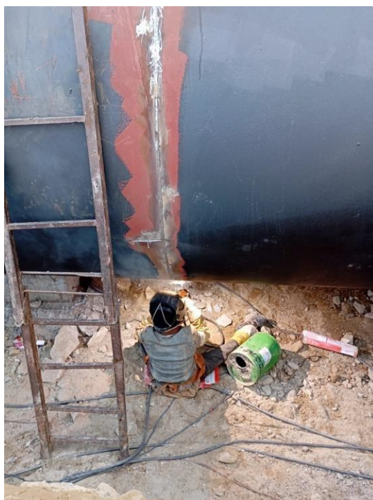
Figure 29: Erection and Painting of pipes
