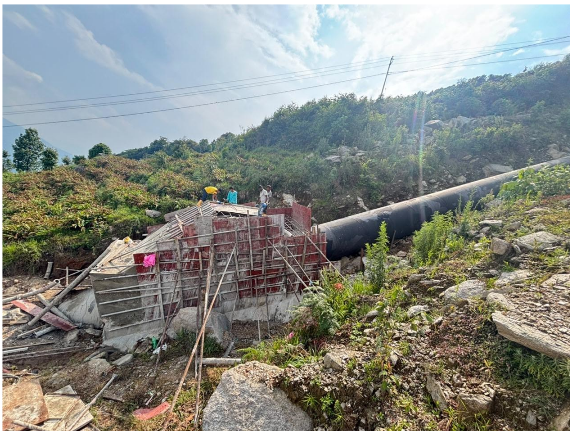
Figure 20: Erection of pipe between and construction of anchor block
