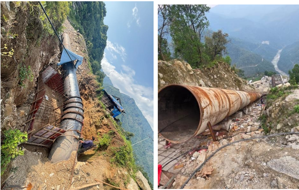
Figure 22: Construction of anchor blocks of penstock pipe
