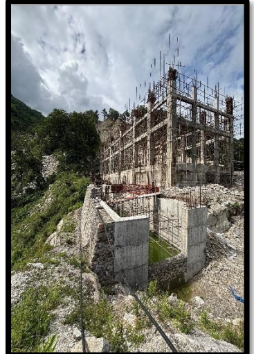
Construction of Cooling P
