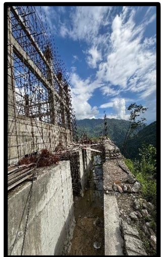
Construction of Tailrace
