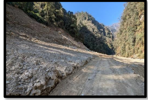
Pondage slope stabilization
