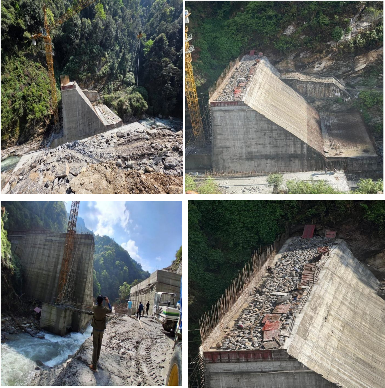
Figure 8: Raised weir along with tower crane
