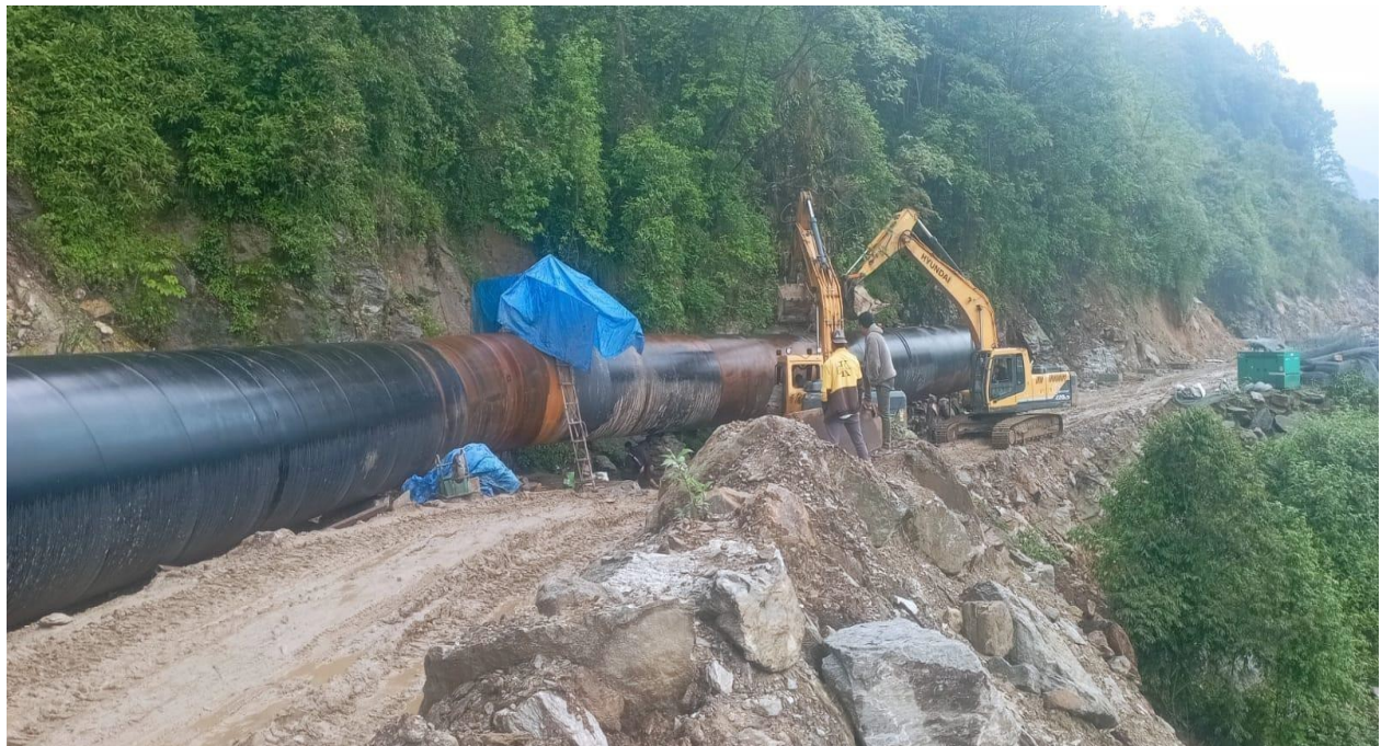
Figure 12: Erection of headrace pipe.
